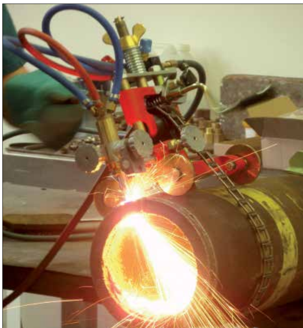
Pipe cutting machine PCM in operation
