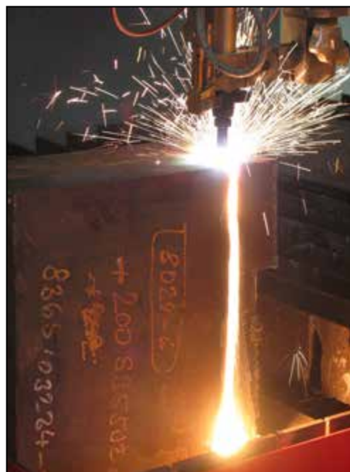
500 mm steel plate cutting
